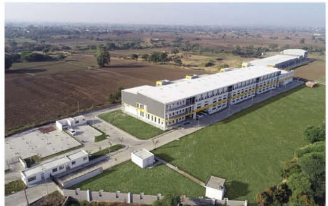
UNIT-3, RAMPLIYA, INDORE
